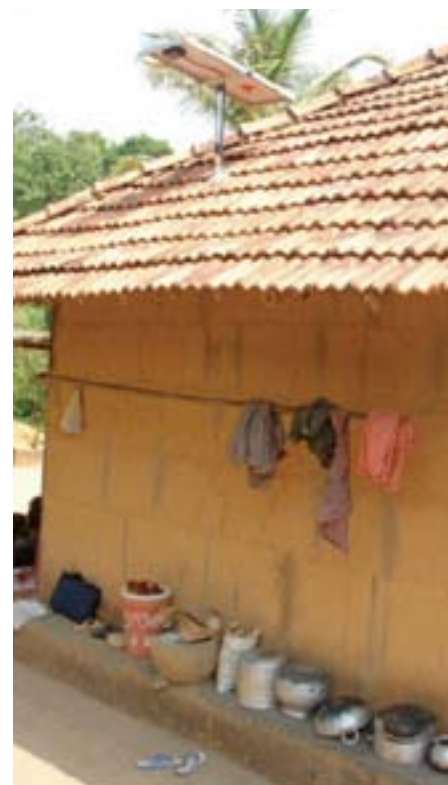
Typical solar light installation in a rural home. Photo: SELCO-India
